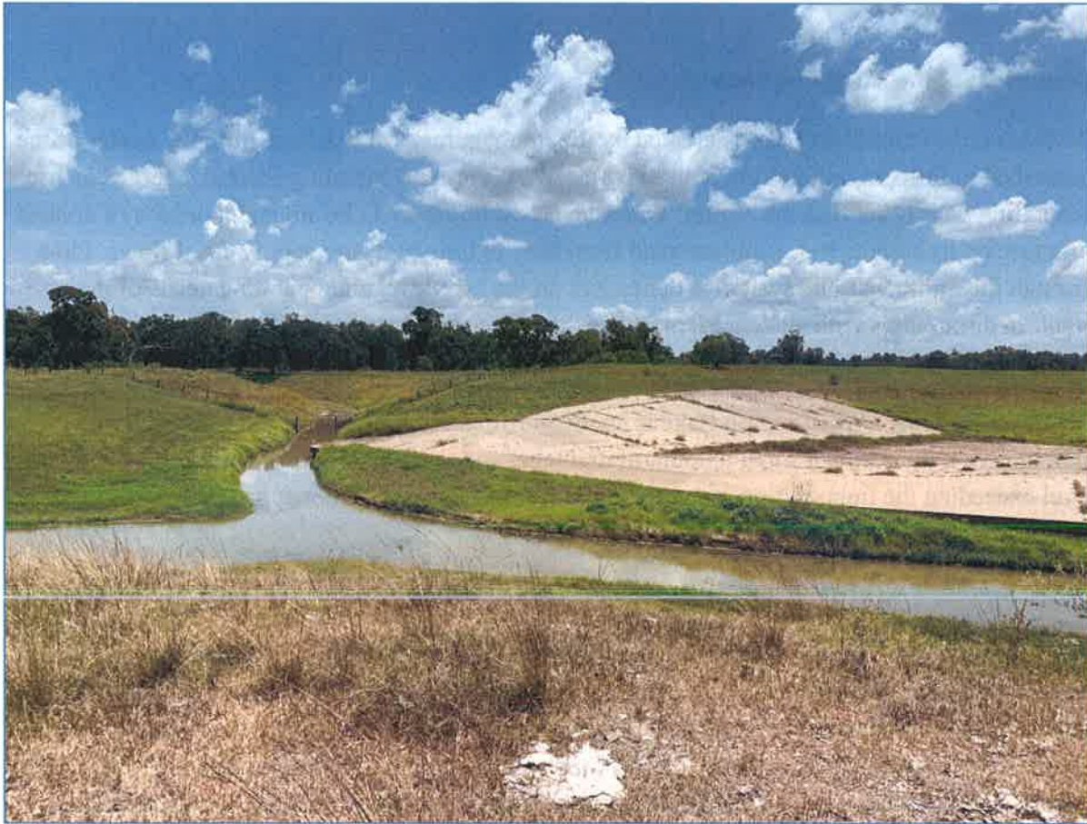
Figure 8 - Drain Bypass Structure at the Confluence of Rabbs Bayou and Big Creek
