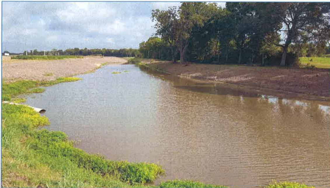
Figure 14 - Stormwater Management Structure near Seabourne Creek Park
